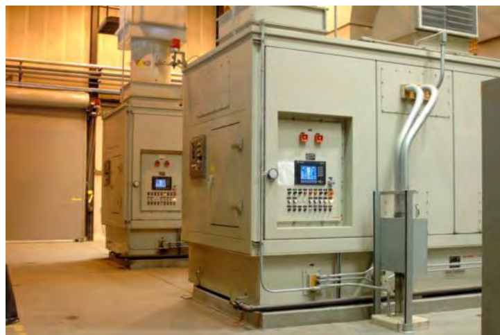
Above, some of the 12 anaerobic digesters. Below, the Solar Centaur-40 gas turbines that turn the biogas into electricity and useful heat.
