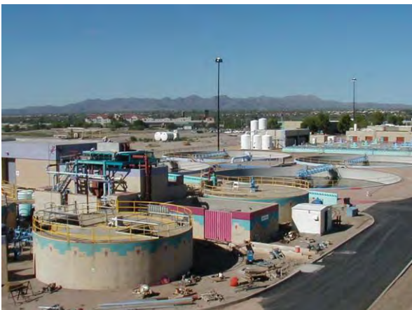
Ina Road Water Pollution Control Facility Tucson, Arizona
