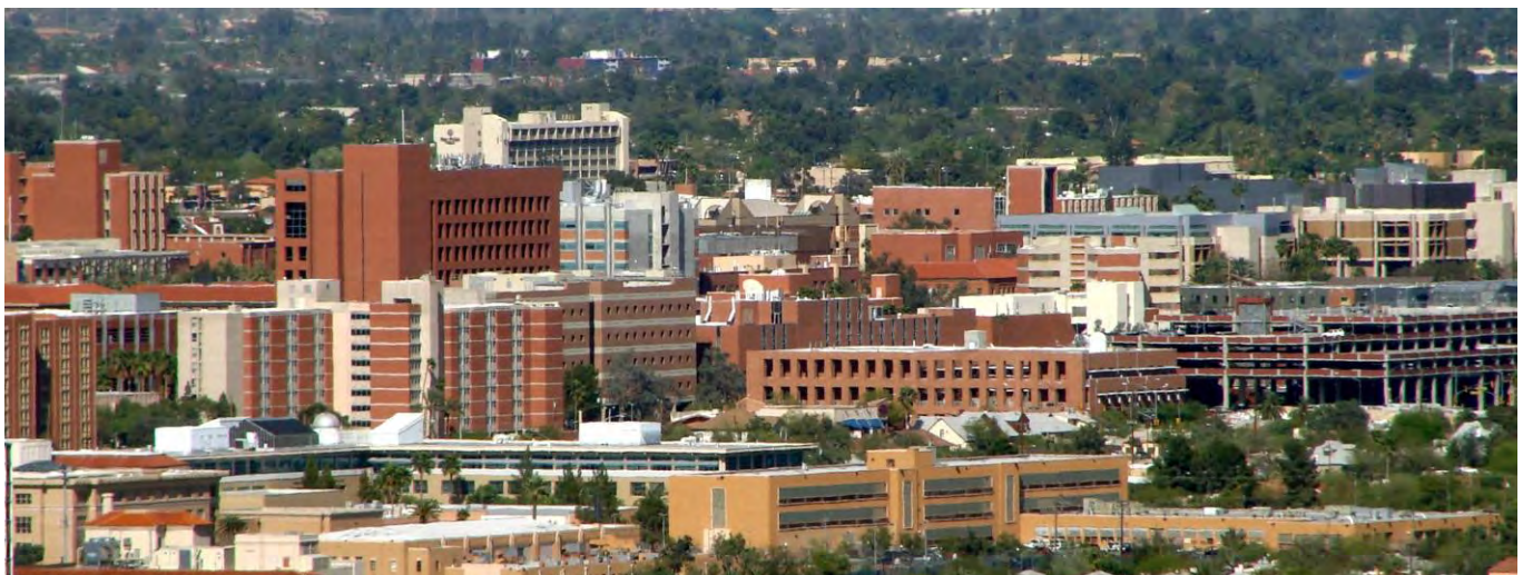
University of Arizona campus in Tucson, Arizona
