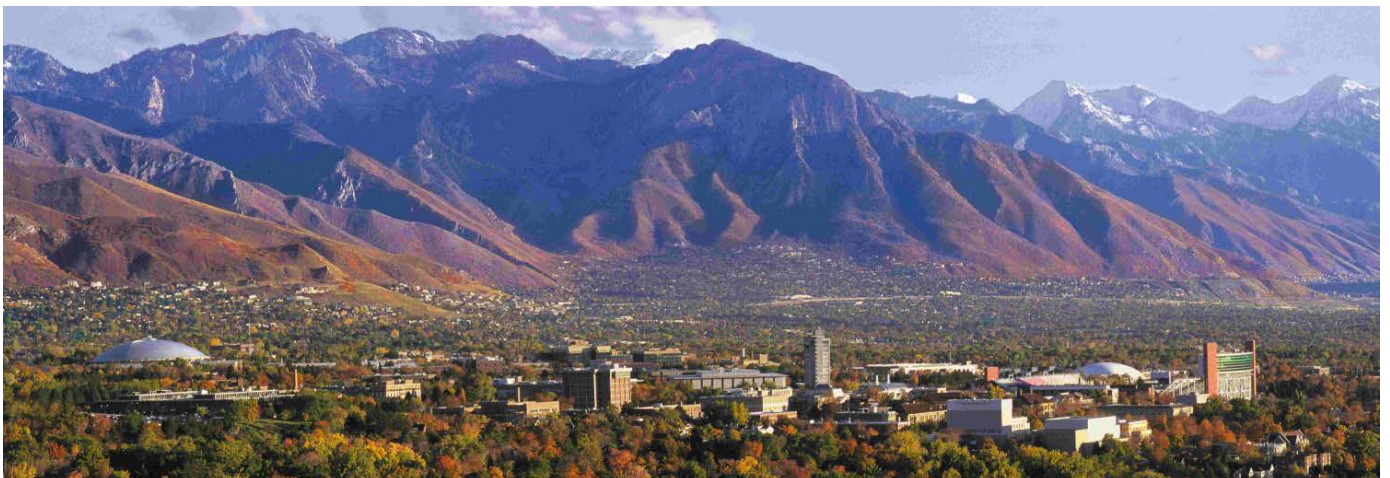
The University of Utah campus in Salt Lake City installed CHP for cost savings and greenhouse gas reductions
